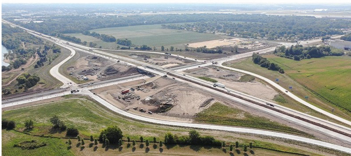
Intersection at Route 2 and Highway 20 in south Rockford.
