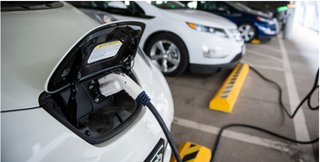
Photo source: U.S. Department of Energy
