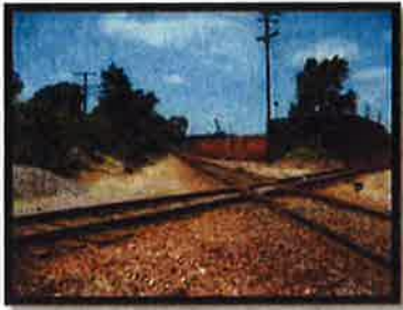
Figure 12 Railroad Diamond Replacement at Buckbee Street
