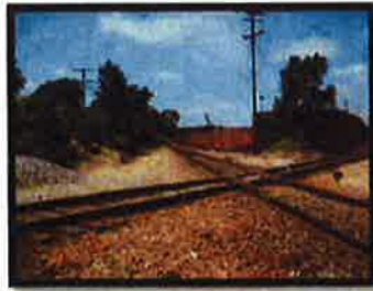
Railroad Diamond Replacement at Buckbee Street
