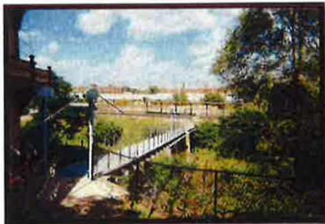
Figure 11 South Main Street Yard
