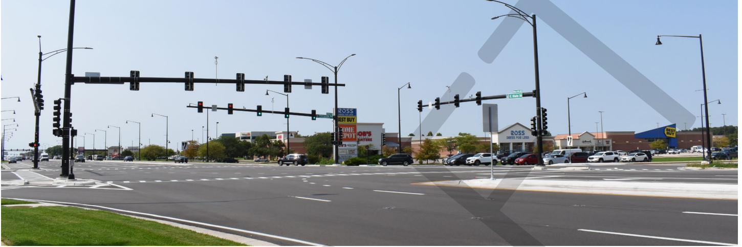
Image 4-3: Principal arterial in Rockford (E State Street)
