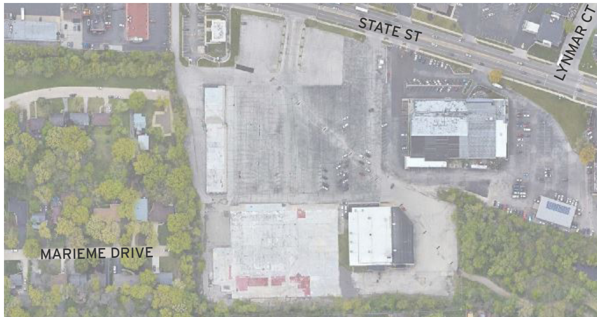
SITE EXISTING CONDITIONS
