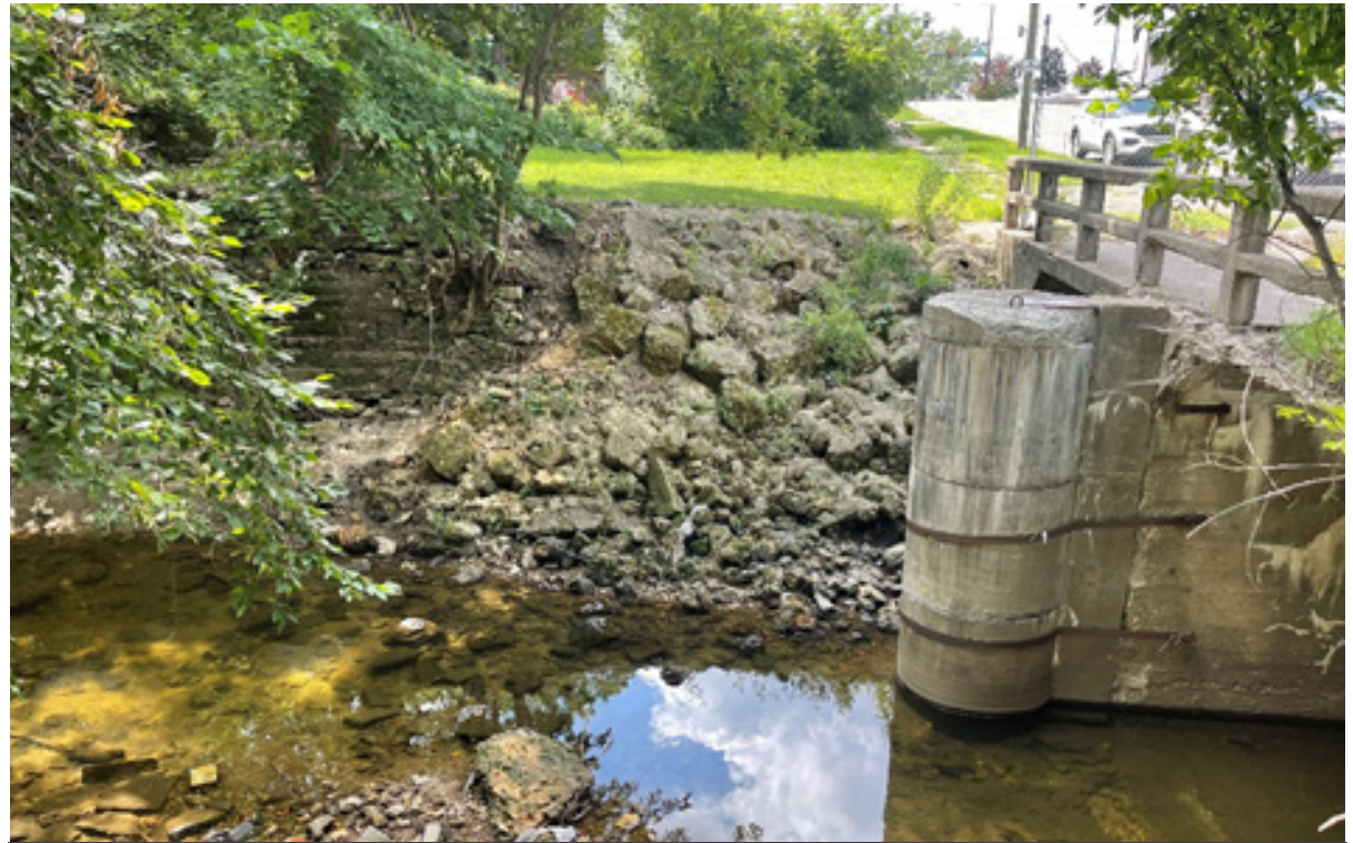
SEWER MANHOLE IN KEITH CREEK
